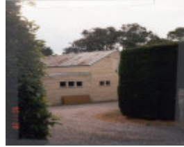
22676 Shed - 245 Tindals Road, Warrandyte (A)
