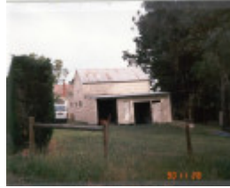
22676 Shed - 245 Tindals Road, Warrandyte (B)
