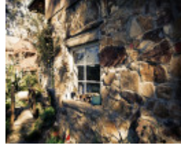
300 Yarra Street, Warrandyte. Stone work detail
