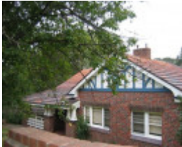
22709 Police Station (former) - 65 Yarra Street, Warrandyte
