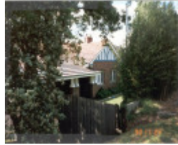
22709 Police Station (former) - 65 Yarra Street, Warrandyte
