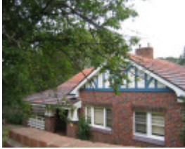
22709 Police Station (former) - 65 Yarra Street, Warrandyte
