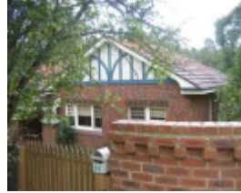
22709 Police Station (former) - 65 Yarra Street, Warrandyte
