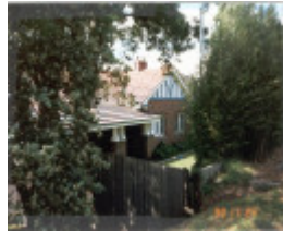
22709 Police Station (former) - 65 Yarra Street, Warrandyte
