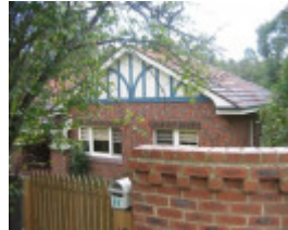
22709 Police Station (former) - 65 Yarra Street, Warrandyte
