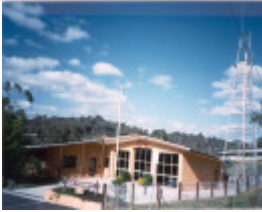
22719 South Warrandyte Fire Station - Brumbys Road, South Warrandyte
