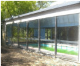
22724 House & internal pool - 138-140 Brysons Road, Warrandyte South (4)
