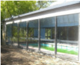
22724 House & internal pool - 138-140 Brysons Road, Warrandyte South (4)
