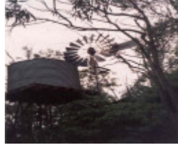
22725 Water Tank - 13 Arunga Road, Wonga Park
