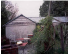
22725 House - 13 Arunga Road, Wonga Park
