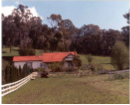
22728 House - 81 Brushy Park Road, Wonga Park
