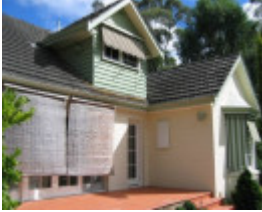
22731 House - 9 Cecil Street, Wonga Park
