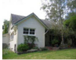
22731 House (rear) - 9 Cecil Street, Wonga Park
