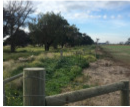
Sub-carrier with concrete outlets - June 2020
