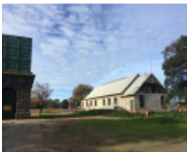
Cocoroc farm hall and Water Tank - June 2020
