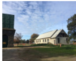
Cocoroc farm hall and Water Tank - June 2020
