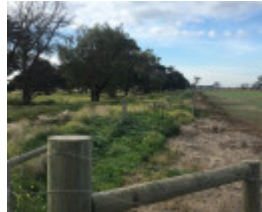
Sub-carrier with concrete outlets - June 2020
