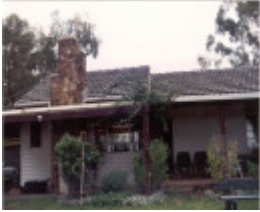
22738 Yarra Brae Cottage - 8 Davis Road, Wonga Park
