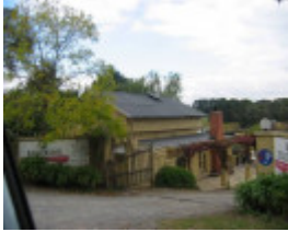
22745 Kellybrook Winery - 1-3 Fulford Road, Wonga Park (8hr village)
