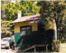
22750 Cottage - 114-116 Jumping Creek Road, Wonga Park
