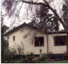
22753 House - 26 Hartley Road, Wonga Park
