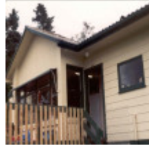
22753 House - 26 Hartley Road, Wonga Park
