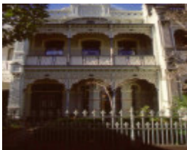
h01831 terrace kerferd rd albert park no33 ac2 june1999
