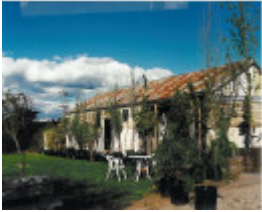
22769 Former Stables - Lower Homestead Road, Wonga Park
