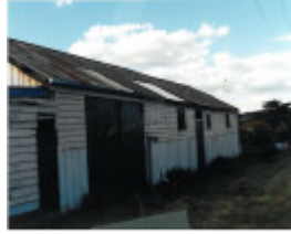
22769 Former Stables - Lower Homestead Road, Wonga Park
