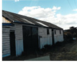
22769 Former Stables - Lower Homestead Road, Wonga Park
