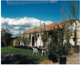
22769 Former Stables - Lower Homestead Road, Wonga Park
