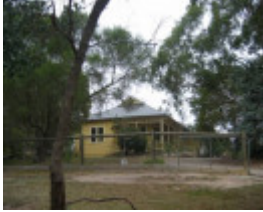
22772 House - 10 Paynters Road, Wonga Park (8hr village)
