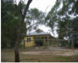
22772 House - 10 Paynters Road, Wonga Park (8hr village)
