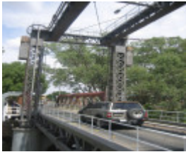
Swan Hill Bridge_Swan Hill_Feb 2008_mz_Lift Span Detail
