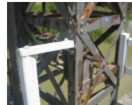
Swan Hill Bridge_Swan Hill_Feb 2008_mz_Winch
