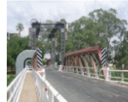
Swan Hill Bridge_Swan Hill_Feb 2008_mz_NSW Approach
