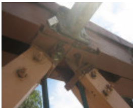
Swan Hill Bridge_Swan Hill_Feb 2008_mz_Truss Connector Detail
