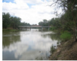
Swan Hill Bridge_Swan Hill_Feb 2008_mz_West Elvation
