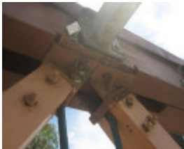
Swan Hill Bridge_Swan Hill_Feb 2008_mz_Truss Connector Detail
