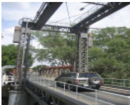
Swan Hill Bridge_Swan Hill_Feb 2008_mz_Lift Span Detail
