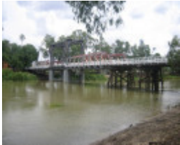
Swan Hill Bridge_Swan Hill_Feb 2008_mz_East Elevation
