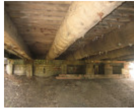
Swan Hill Bridge_Swan Hill_Feb 2008_mz_Round Timber Girders
