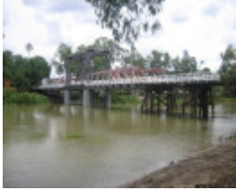
Swan Hill Bridge_Swan Hill_Feb 2008_mz_East Elevation
