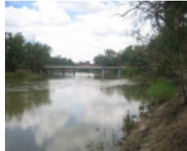
Swan Hill Bridge_Swan Hill_Feb 2008_mz_West Elvation
