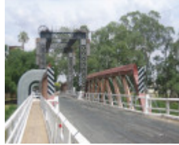
Swan Hill Bridge_Swan Hill_Feb 2008_mz_NSW Approach
