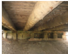
Swan Hill Bridge_Swan Hill_Feb 2008_mz_Round Timber Girders
