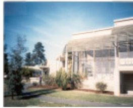
22961 Box Hill TAFE (Former) - Deep Creek Drive, Doncaster East (2)
