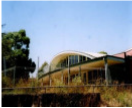
22961 Box Hill TAFE (former) - Deep Creek Drive, Doncaster East (1)
