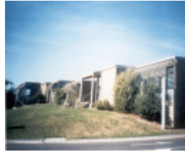
22961 Box Hill TAFE (former) - Deep Creek Drive, Doncaster East (3)
