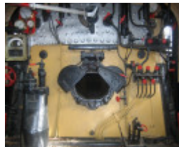
Heavy Harry_Loco H220_ARHS Museum Newport_2 May 2007_Firebox and Mechanical Stoker
