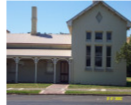
23063 Wannon Shire Offices Coleraine 0428
