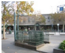
H2111 Underground Toilets Elizabeth & Victoria Sts 08 06 06 mz 001
