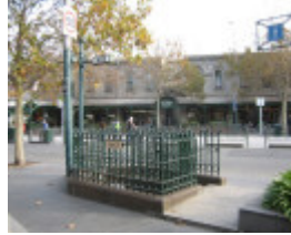
H2111 Underground Toilets Elizabeth & Victoria Sts 08 06 06 mz 001
