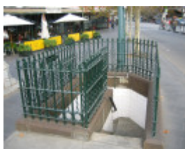
H2111 Underground Toilets Elizabeth & Queen Sts 08 06 06 mz 011
