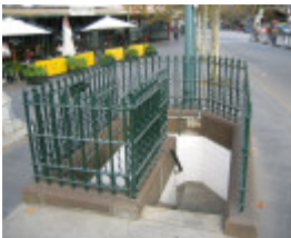
H2111 Underground Toilets Elizabeth & Queen Sts 08 06 06 mz 011
