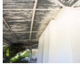
H0361 Kongbool verandah roof 2379
