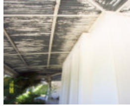
H0361 Kongbool verandah roof 2379
