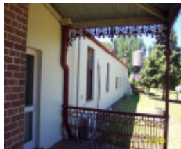
23123 Englefield Balmoral north verandah 2305
