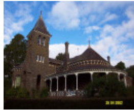
H0541 Kolor Penshurst entrance tower 0845
