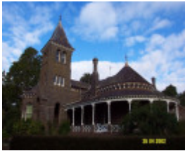
H0541 Kolor Penshurst entrance tower 0844
