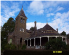
H0541 Kolor Penshurst entrance tower 0844
