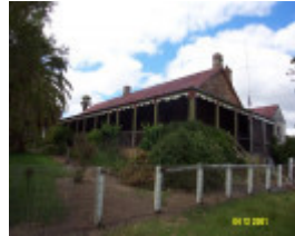
23132 Clunie Homestead front verandah 0271
