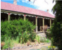
23132 Clunie Homestead front verandah 0270
