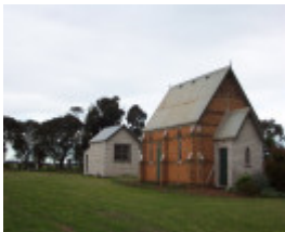
23140 Zion Lutheran Church Byaduk 0077
