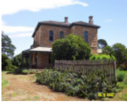
H1925 Gringegalgonia Homestead facade 2207
