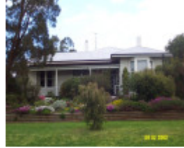
23166 Hospital Former 99 McKebery St Coleraine 1509
