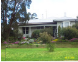
23166 Hospital Former 99 McKebery St Coleraine 1508
