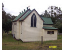
23170 Catholic church rear view Harrow 0276
