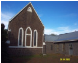
23176 St Andrews Uniting Church Penshurst rear 0853
