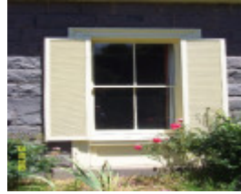
23187 Warrayure Homestead Complex window 1884
