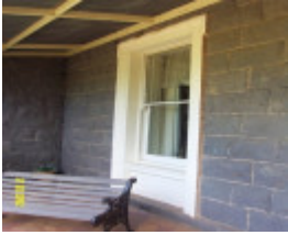
23187 Warrayure Homestead Complex window 1876
