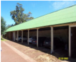
23187 Warrayure Homestead Complex machinery shed 1889
