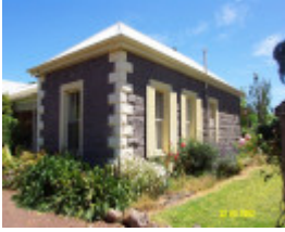
23187 Warrayure Homestead Complex side windows 1882
