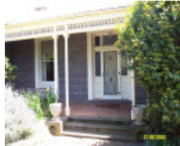
23187 Warrayure Homestead Complex front door 1877
