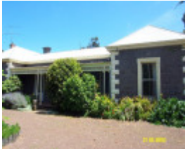
23187 Warrayure Homestead Complex facade 1878
