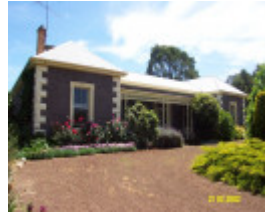
23187 Warrayure Homestead Complex facade 1879
