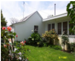
23188 Brung Brungle rear of outbuildings 0196
