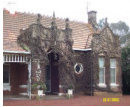
23192 Bassett Homestead Branxholme front elevation 1406
