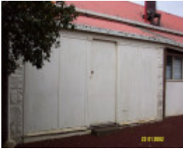
23192 Bassett Homestead Branxholme rear elevation 1416
