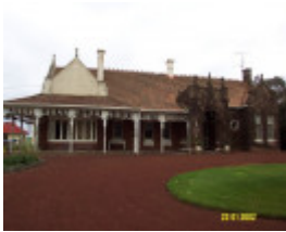
23192 Bassett Homestead Branxholme front elevation 1405
