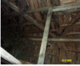
23192 Bassett Homestead Branxholme tank stand 1401
