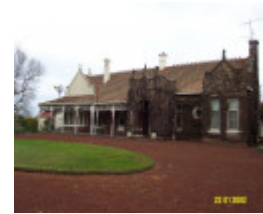
23192 Bassett Homestead Branxholme front elevation 1407
