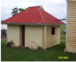
23192 Bassett Homestead Branxholme dairy 1395
