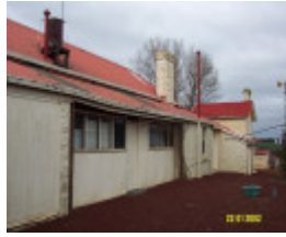
23192 Bassett Homestead Branxholme rear elevation 1417
