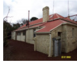
23192 Bassett Homestead Branxholme rear elevation 1418
