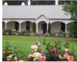
23195 Nareen Homestead Complex facade 1926
