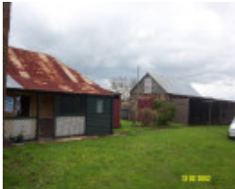
23199 Victoria Hotel Former 100 Bell St Penshurst 1522
