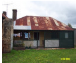
23199 Victoria Hotel Former 100 Bell St Penshurst 1524
