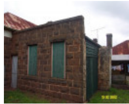
23199 Victoria Hotel Former 100 Bell St Penshurst 1523
