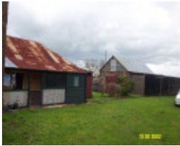
23199 Victoria Hotel Former 100 Bell St Penshurst 1522
