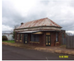
23199 Victoria Hotel Former 100 Bell St Penshurst 1521
