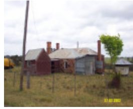
23205 Springwood Homestead Wannan stone cottage 2064
