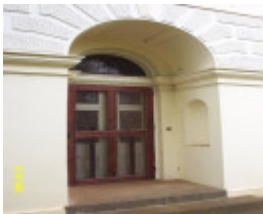
23205 Springwood Homestead Wannan entrance 2049
