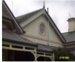
23205 Springwood Homestead Wannan gable detail 2051
