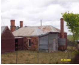
23205 Springwood Homestead Wannan stone cottage 2063
