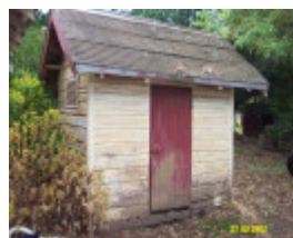
23205 Springwood Homestead Wannan split timber outbuilding 2072
