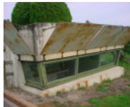
h01090 fort franklin portsea bunker observation post 01 0604 js
