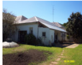
23221 Koornong Homestead kitchen 0699
