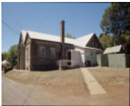
Christ Church School_Daylesford_South Elevation_Feb 2004_mz
