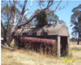
23254 Timber Kiln and Boiler Balmoral 2095
