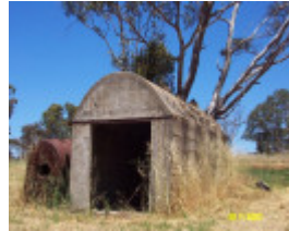
23254 Timber Kiln and Boiler Balmoral 2096
