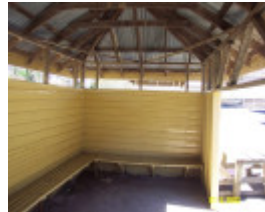
23257 Consolidated School Balmoral shelter 2179
