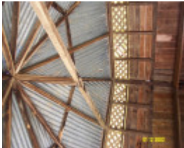
23257 Consolidated School Balmoral shelter 2178
