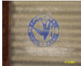
23257 Consolidated School Balmoral shelter 2180
