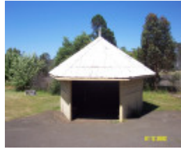
23257 Consolidated School Balmoral shelter 2177
