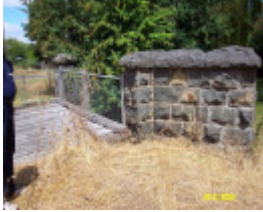
23277 Bluestone Mill Bridge Byaduk 0387
