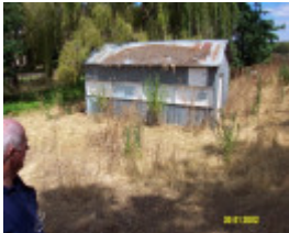
23286 Swimming Pool Byaduk kiosk 0386
