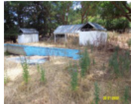
23286 Swimming Pool Byaduk shelter shed 0385
