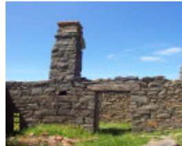
23288 Albert Homestead complex house 1860
