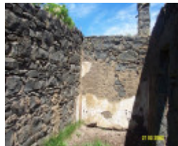
23288 Albert Homestead complex house 1864
