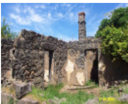
23288 Albert Homestead complex house 1865
