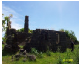
23288 Albert Homestead complex house 1861
