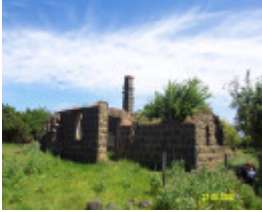
23288 Albert Homestead complex house 1862
