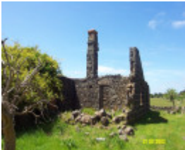
23288 Albert Homestead complex house 1859
