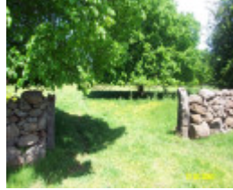
23288 Albert Homestead complex gateway 1874
