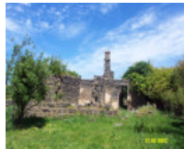
23288 Albert Homestead complex house 1863
