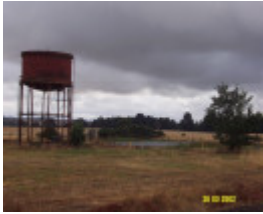
23291 Railway Water tower Branxholme 0559
