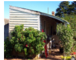
23304 Brae Park Branxholme shed 0722
