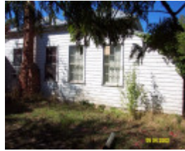
23310 Timber House Branxholme 0717
