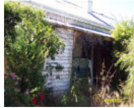
23310 Timber House Branxholme 0715
