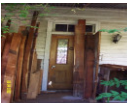
23310 Timber House Branhholme verandah 0720
