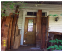
23310 Timber House Branxholme verandah 0720
