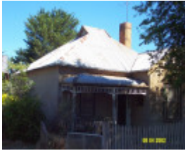
23310 Timber House Branxholme 0710
