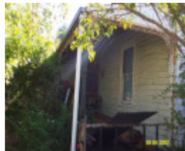
23310 Timber House Branxholme verandah 0718
