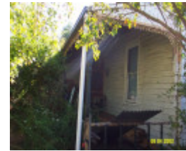
23310 Timber House Branhholme verandah 0718
