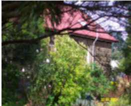
23325 Wesley Ch Former 77 Bell St Penshurst 0788
