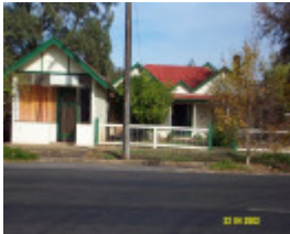
23327 Common School Former 83a b Bell St Penshurst 0804
