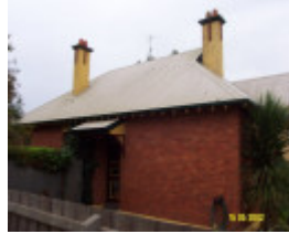
23332 Police Residence Martin St Penshurst S side 1005
